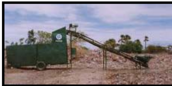
Mobile sieving machine in dumping yard
