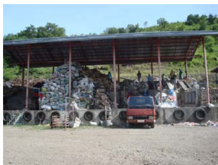
MRF station at San Carlos Eco-center
