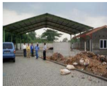
Material Recovery Facility of BEST
