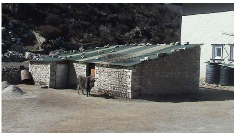
Biogas plant in Mountain region of Nepal
