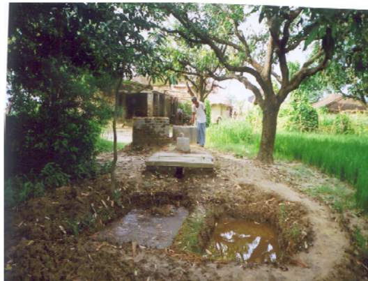
Biogas plant in Terrain region of Nepal
