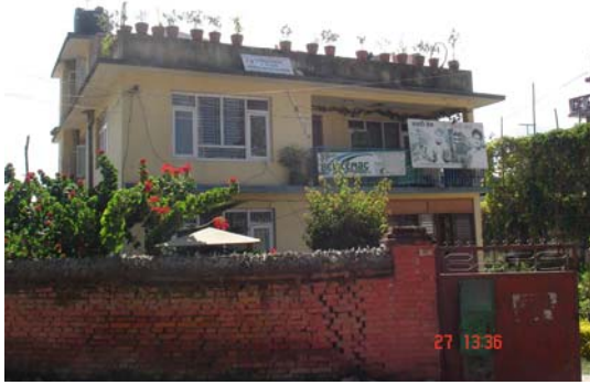
NEPCEMAC Head Office
